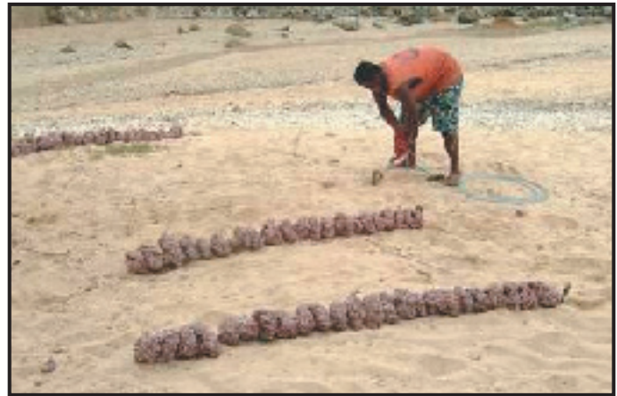
Figure 12: Rock substrate strung together using galvanized wire
