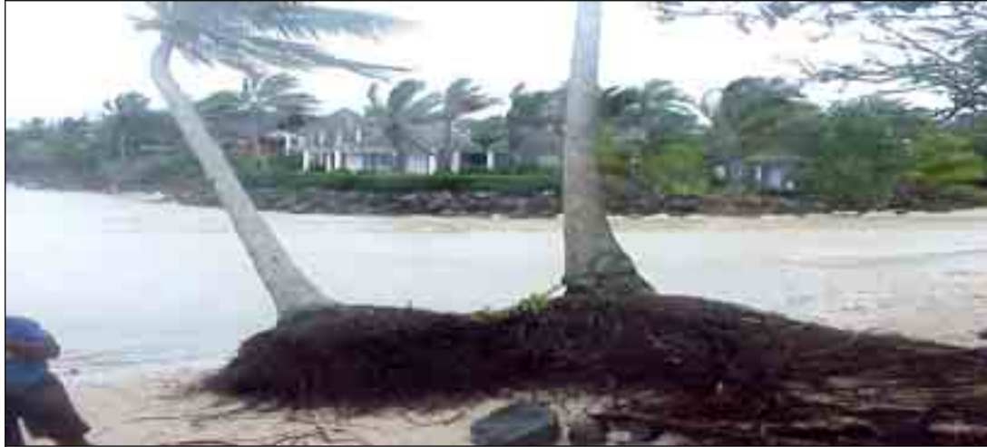
Photograph 2. Rock revetments in the background have resulted in the degradation of adjacent properties.
