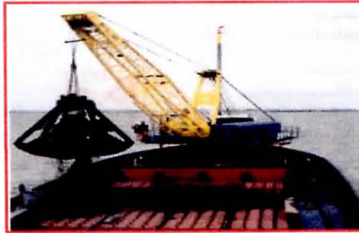
Figure 54. Example of the crane to be used by the dredge ship.
