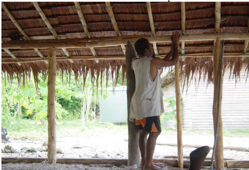
Plate 4 House construction in process
