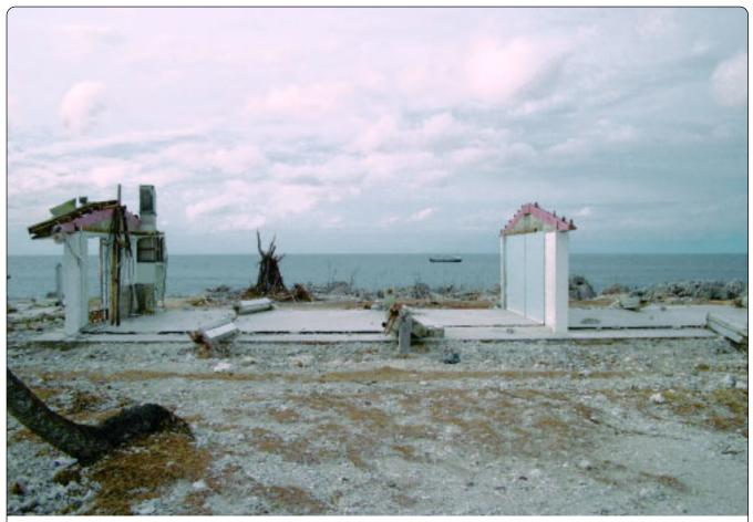
Cyclone Heta, which struck Niue in January 2004, was a category 5 cyclone. This duplex building was 85 m landward of the cliff face. Severe damage also occurred in Samoa, Tokelau and Tonga
