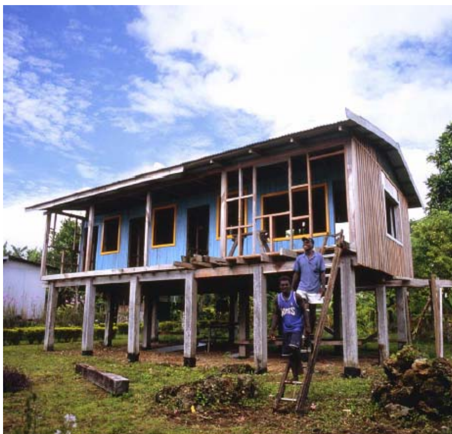
Figure 3: IWP building under construction in Chea, Marovo Lagoon, Solomon Islands
