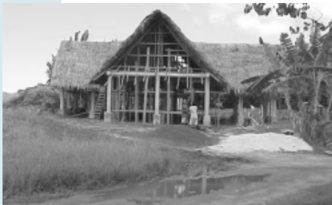
Construction well under way on the Utwa–Walung Centre
