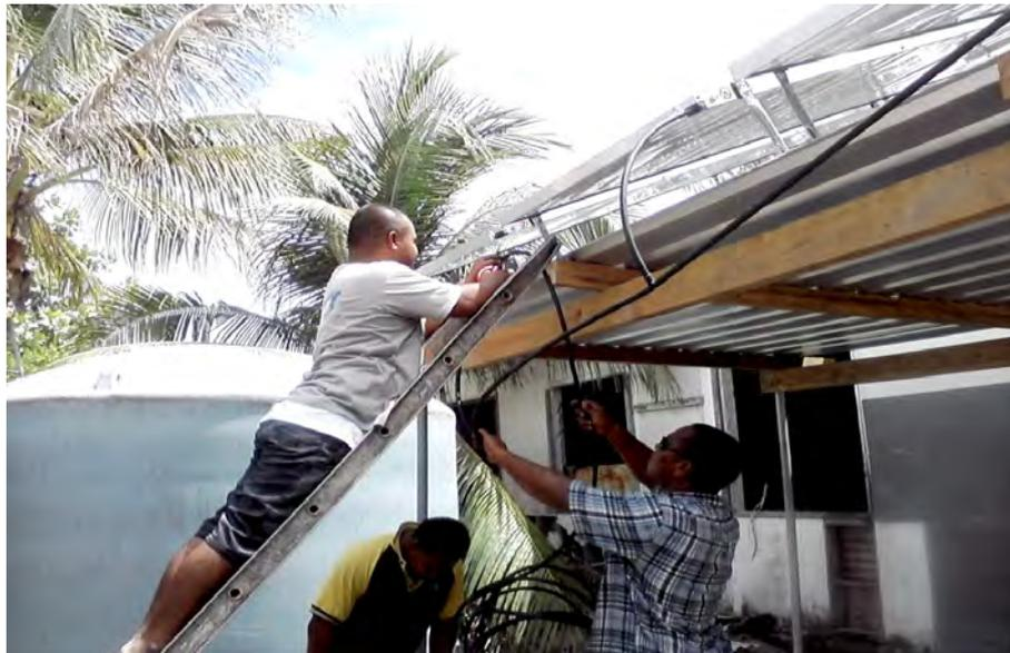
Figure 8. Installing solar panels on a platform designed for householders in Aiwo district (photo: PACC Nauru).
