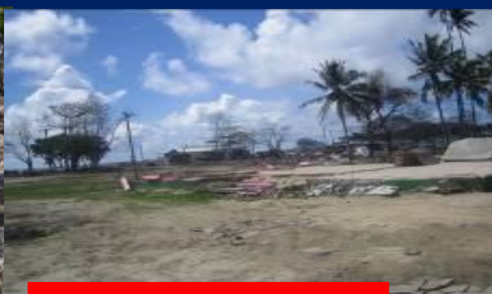
After DWM Project
