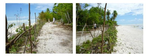
**Figure 9.** Site 1b at Tabon-ke-bike in October 2013, after the brush wave barrier was made more substantial, and the read edge was fenced to control disturbance.
