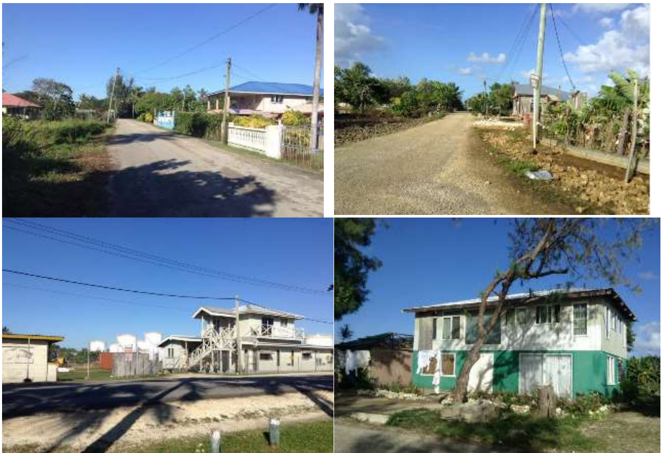
Photo 4: Typical Conditions in Area 4
