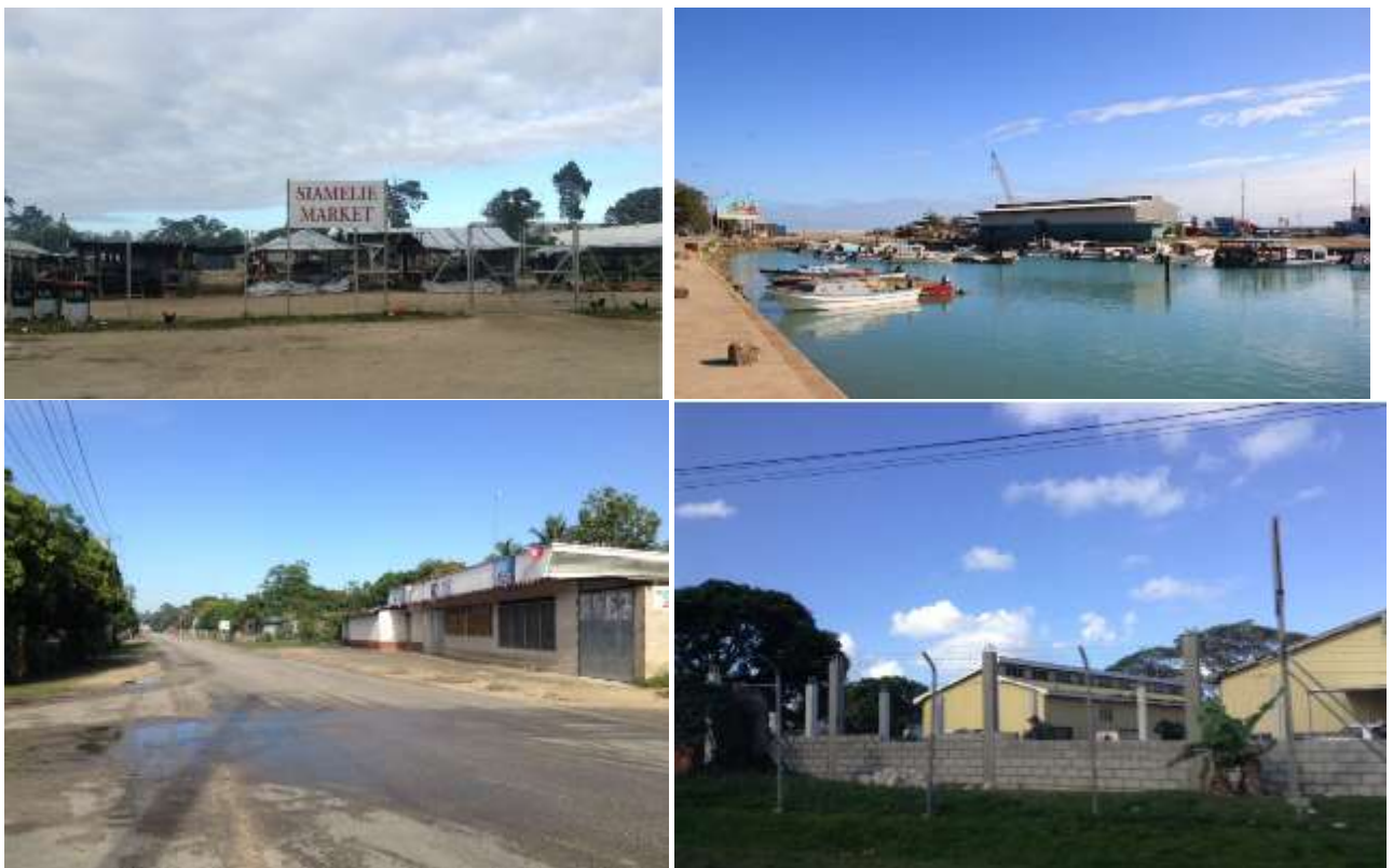
Photo 3: Typical Conditions in Area 3
