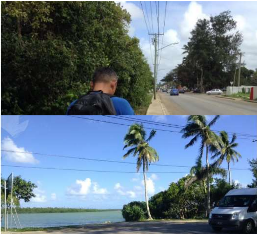
Photo 12: Distribution line closest to the shoreline of Fanga'uta and Fangakakau Lagoon Marine Sanctuary
