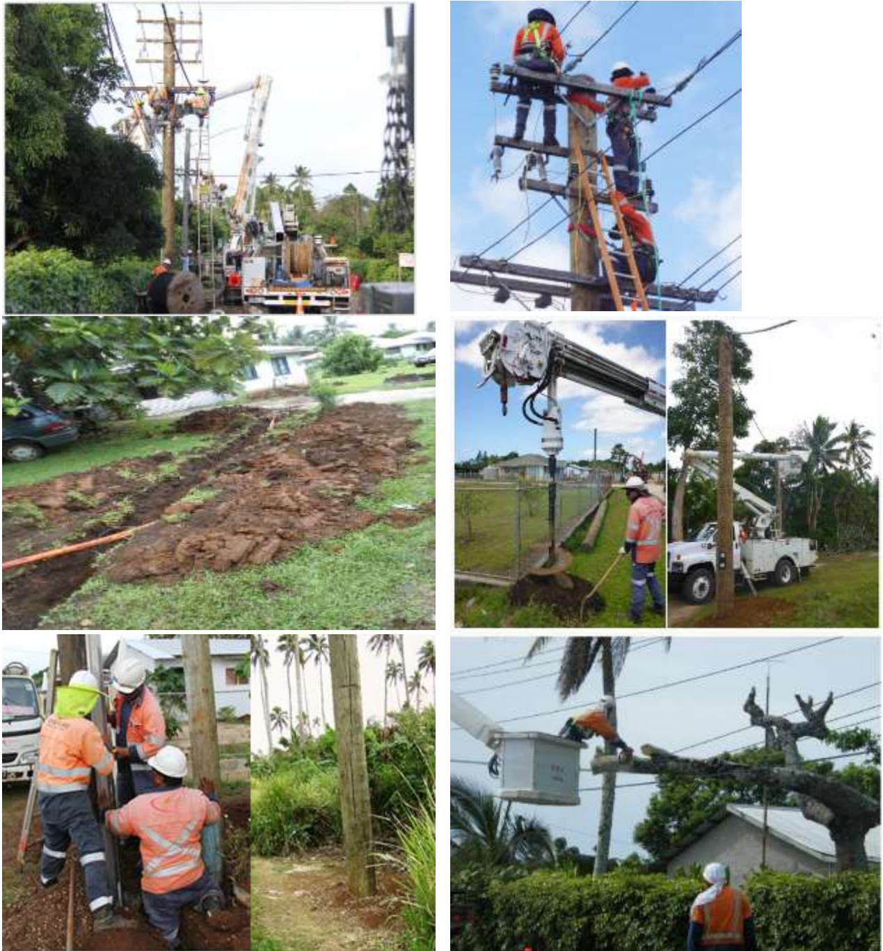
Photo 11: Typical Work on the Distribution Lines
