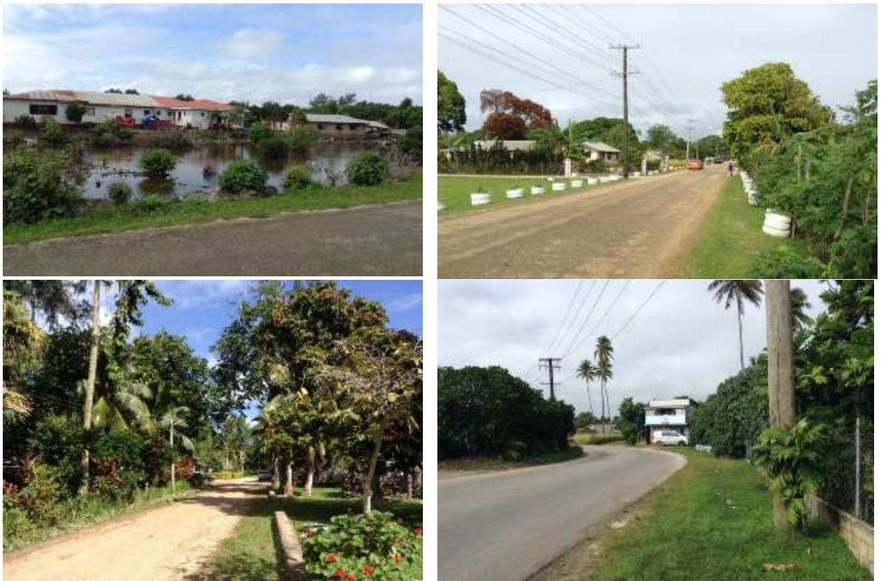
Photo 5: Typical Conditions in Area 5
