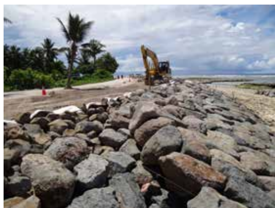
Rock revetment at South Tarawa, Kiribati
