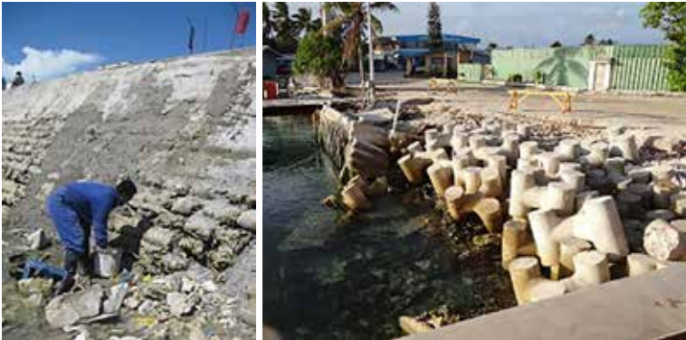
Figure 6-12 Examples of seawall repair
