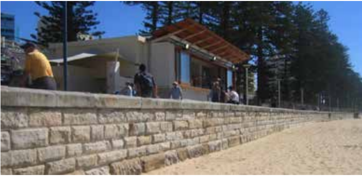
Figure 3-2 Example of a Rigid Vertical Seawall
