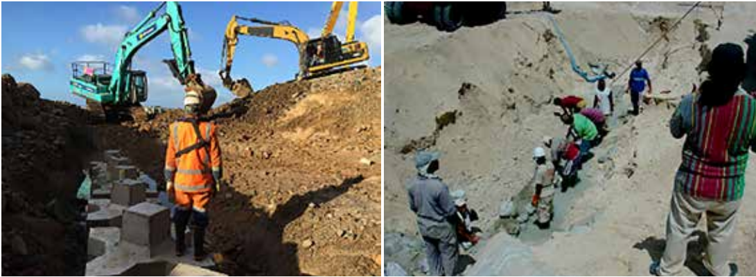
Figure 6-8 Example of revetment toe excavation
