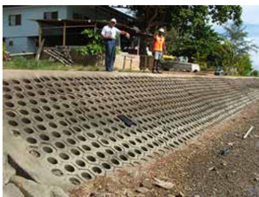
Seabee seawall Boigu Island, Torres Strait (Source: P. Riedel, 2005)
