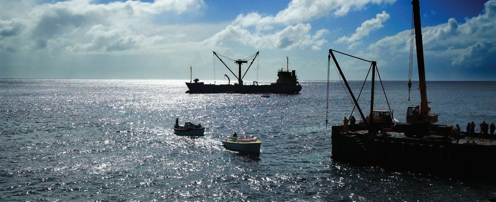
All goods shipped to Norfolk Island are unloaded offshore and brought ashore by a smaller boat. This provides some protection against hitchhiker organisms on ships making it to shore. A new wharf is being built that will allow ships to moor alongside – one of many ways in which biosecurity risks are changing on Norfolk Island. Photo: thinboyyfatter | Flickr | CC BY 2.0
