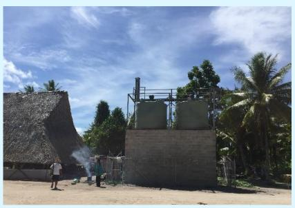
Photo 3.2: KAP-III rainwater harvesting scheme in North Tarawa, Kiribati
