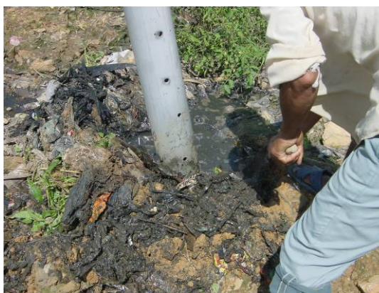
Photo- 44: Clogged Vertical Gas Venting Pipes
