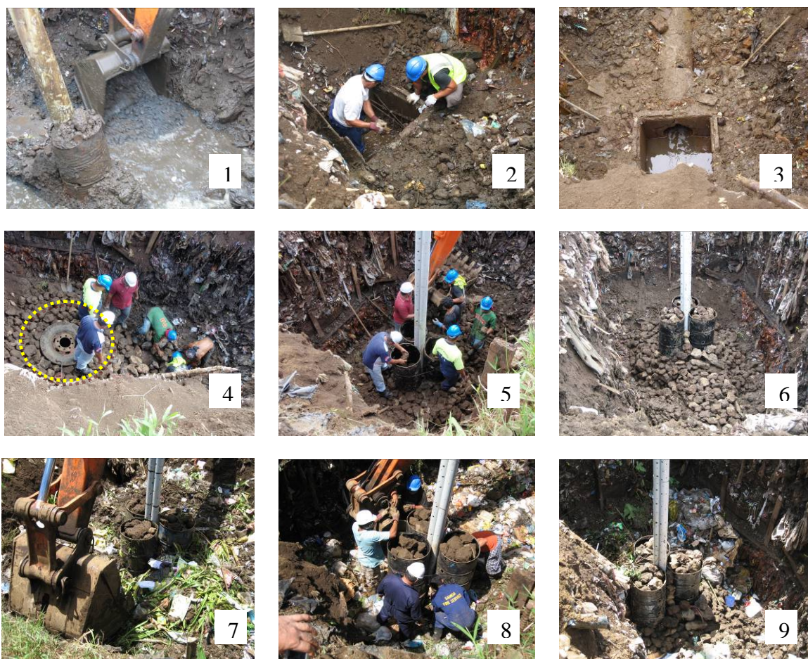
Photo- 45: Sequence of Remediation of Damaged Gas Venting Facility on the Connection Pit
