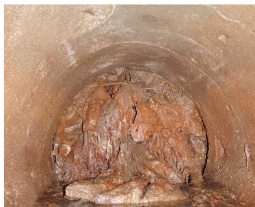
Photo- 43 Clogged Leachate Collection Pipes
