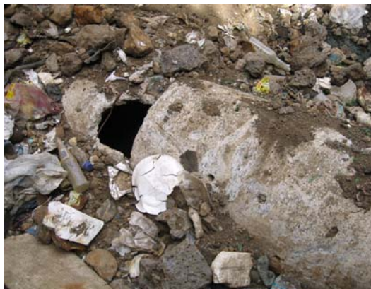
Photo- 42: Damaged Leachate Collection Pipes
