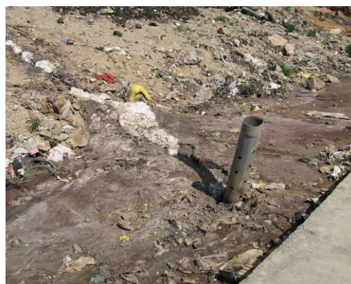
Photo- 44: Clogged Vertical Gas Venting Pipes
