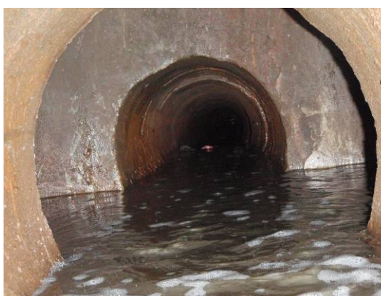
Photo- 43 Clogged Leachate Collection Pipes
