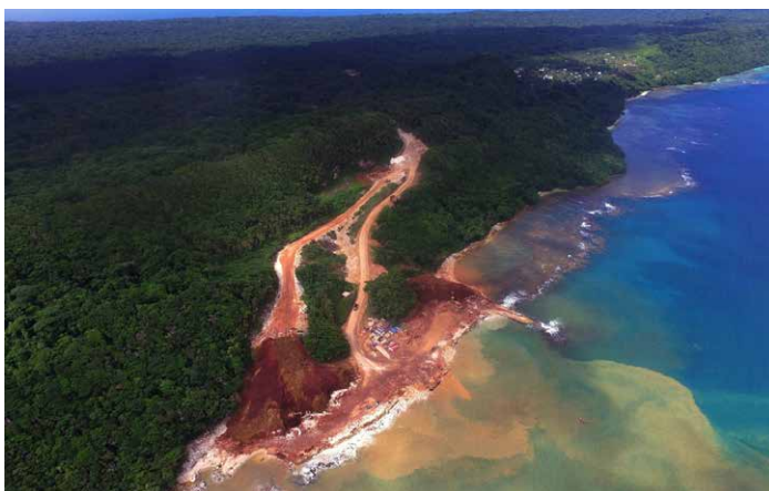
FIGURE 3.23. BMSI Lavangu port terminal, Rennell Island (©Edward Danitofea, MECDM)
